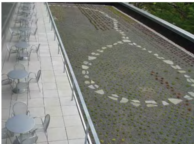
This recently planted green roof on top of the FedEx Global Education Center will manage stormwater and provide an attractive view from the fourth floor patio.
