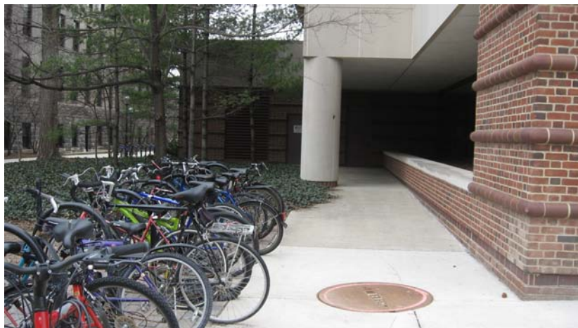
Figure 2. Chemistry Building East Side
