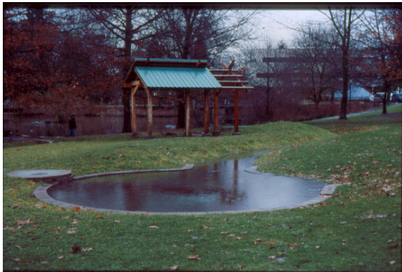
Fig. 4 Bioswale earthwork, University of Oregon
