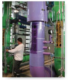
The chilled water plant and its 2.6 million gallon storage tank enables the University to purchase electricity at a lower cost to operate chillers during non-peak evening hours and store the chilled water for use during the day for air conditioning campus buildings and cooling specialized laboratory equipment.
